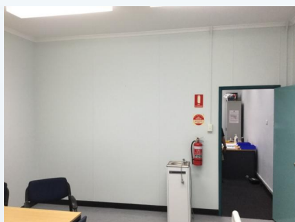
NO.: 14 PHOTO NO.: J159257-NT0557A-PHOTO018 RESULT: ASBESTOS - PREVIOUSLY SAMPLED POSITIVE BUILDING/LEVEL: NIGHTCLIFF POLICE STATION - GROUND LEVEL ROOM/LOCATION: STAFF LUNCH ROOM - NORTH FEATURE/MATERIAL: WALL LINING - FIBRE CEMENT SHEETING SAMPLE NO.: PREVIOUSLY SAMPLED AEC AS PER 5-3013
