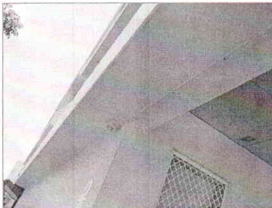
Photo 2, Lining to underside of cladding overhang
