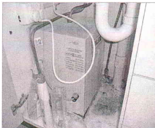
Photo 6. Wire insulation to HWS in lunchroom
