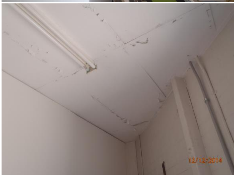
Photograph 14 AC ceiling tiles throughout Shop 8 (assumed asbestos containing).
