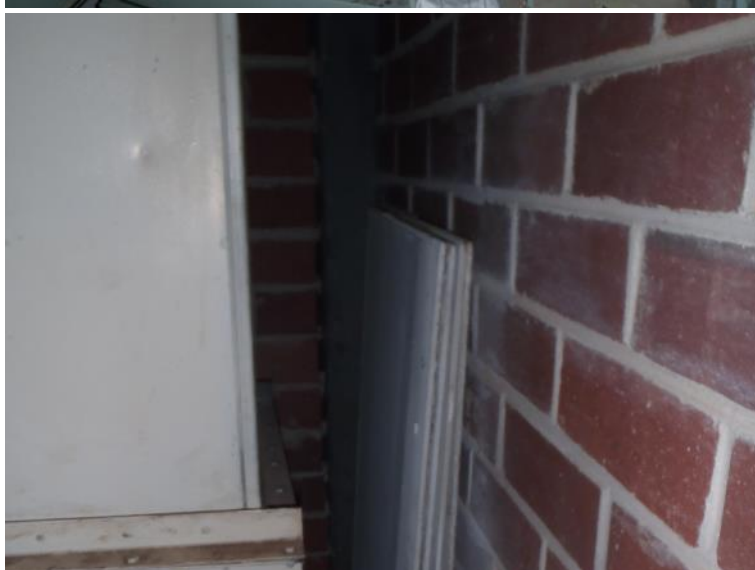
Photograph 48 Loose AC ceiling tiles stored behind AC ducting to upper plant room off Shop 28A (assumed asbestos containing).
