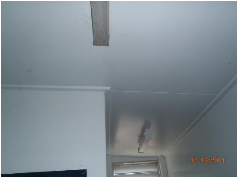
Photograph 61 AC sheeting ceiling to Male public toilets (asbestos containing).
