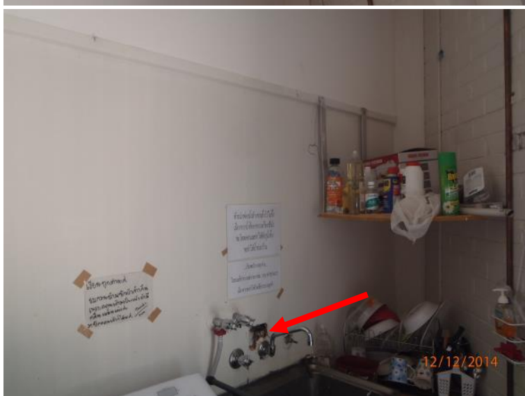
Photograph 15 AC sheet to lower wall lining to laundry area of Shop 8 – note damage around tap (assumed asbestos containing).
