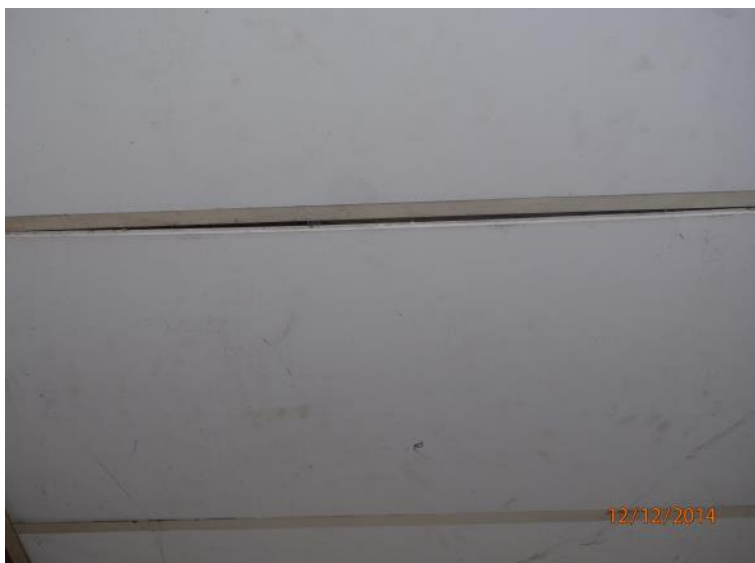
Photograph 46 AC ceiling tiles throughout Shop 28 (assumed asbestos containing).
