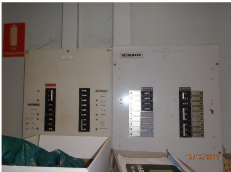
Photograph 13 Backing boards to electrical boxes in Shop 7 (assumed asbestos containing).
