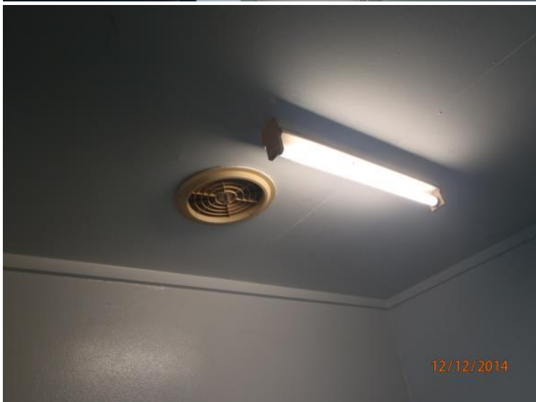
Photograph 62 AC sheeting ceiling to female public toilets (assumed asbestos containing).
