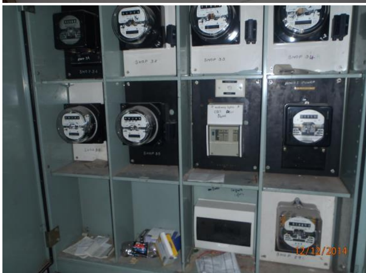
Photograph 47 Backing boards to electrical boxes (x 2) to Shop 28 (Power Room 1) (assumed asbestos containing).
