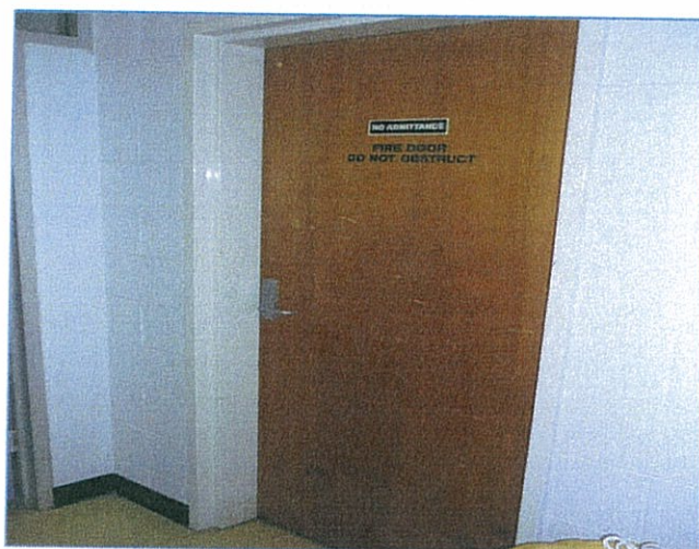
Photo 8 Fire door to entry of AC plant room
