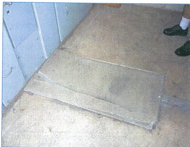
Photo 20 Cement sheet covers to sub floor area of Sub Station area
