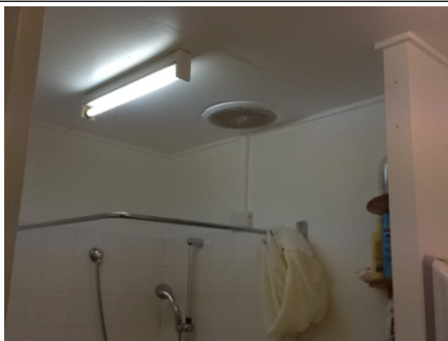
Photo No: j119922-NT0554-333 Result: Asbestos - Presumed Positive Building/Level: Main Building - Anglicare-Ground Level Room/Location: Female Toilets-Throughout Feature/Material: Ceiling-Insulating Board
