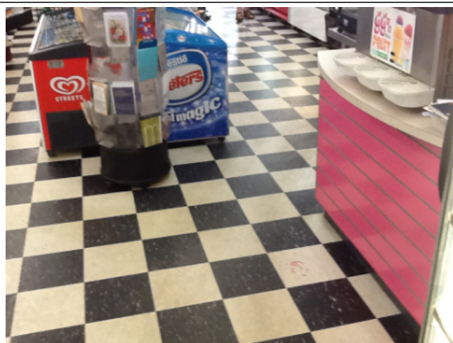
Photo No: j119922-NT0554-319 Result: Asbestos - Positive Building/Level: Main Building - Supermarket-Ground Level Room/Location: Store floor-Throughout Feature/Material: Floor Covering-Vinyl Tiles & Adhesive
