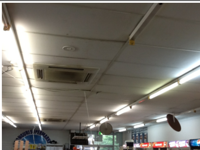
Photo No: j119922-NT0554-321 Result: Asbestos - Positive Building/Level: Main Building - Supermarket-Ground Level Room/Location: Retail area-Throughout Feature/Material: Ceiling Tiles-Compressed Cement Sheet
