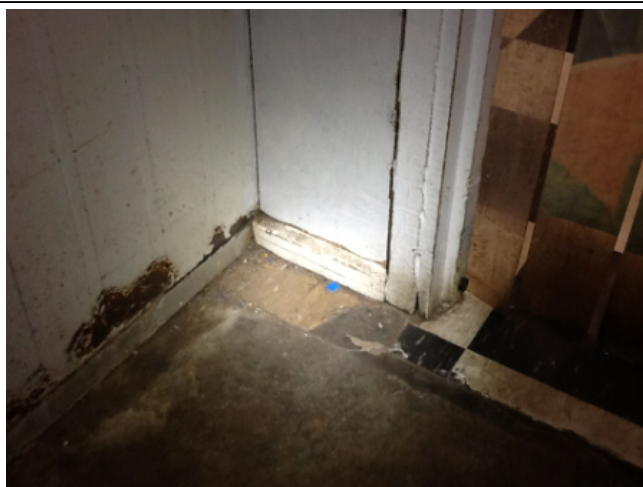
Photo No: j119922-NT0554-320 Result: Asbestos - Positive Building/Level: Main Building - Supermarket-Ground Level Room/Location: Storage Room-Adjacent to store entry door Feature/Material: Floor Covering Adhesive-Vinyl Tiles & Adhesive
