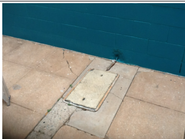
Photo No: j119922-NT0554-338 Result: Asbestos - Positive Building/Level: Main Building - Darwin Midwifery Group-Ground Level Room/Location: Exterior-East Feature/Material: Pit-Moulded Fibre Cement
