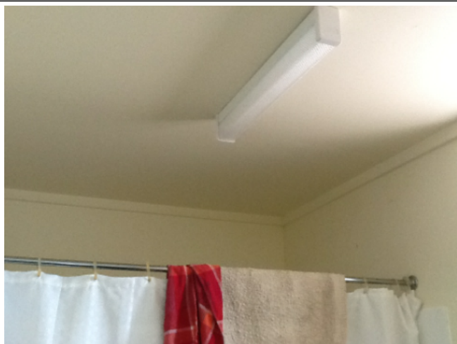
Photo No: j119922-NT0554-336 Result: Asbestos - Presumed Positive Building/Level: Main Building - Anglicare-Ground Level Room/Location: Meeting room toilets-Throughout Feature/Material: Ceiling-Insulating Board
