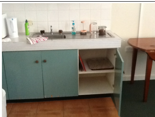
Photo No: j119922-NT0554-337 Result: Asbestos - Positive Building/Level: Main Building - Anglicare-Ground Level Room/Location: Meeting Room-Below sink Feature/Material: Sink Lining-Bituminous Material
