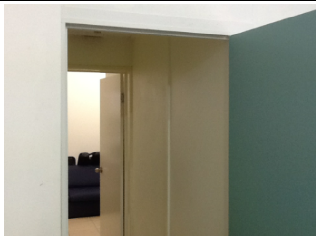
Photo No: j119922-NT0554-330 Result: Asbestos - Positive Building/Level: Main Building - Anglicare-Ground Level Room/Location: Connecting passage-South Feature/Material: Wall Lining-Compressed Cement Sheet
