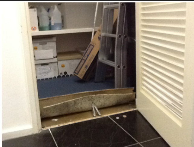
Photo No: j119922-NT0554-334 Result: Asbestos - Positive Building/Level: Main Building - Anglicare-Ground Level Room/Location: Storage Cupboard-Throughout Feature/Material: Floor Covering-Vinyl Tiles & Adhesive
