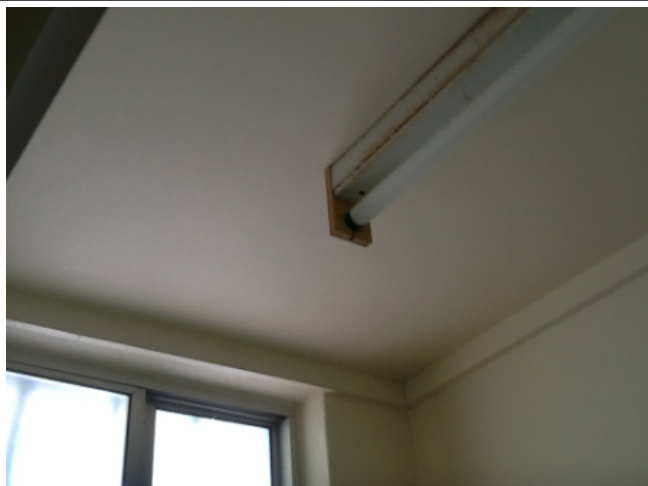
Photo No: j119922-NT0554-328 Result: Asbestos - Presumed Positive Building/Level: Main Building - Anglicare-Ground Level Room/Location: Toilets-Throughout Feature/Material: Ceiling-Insulating Board
