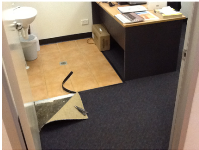
Photo No: j119922-NT0554-326 Result: Asbestos - Positive Building/Level: Main Building - Darwin Midwifery Group-Ground Level Room/Location: Consult Room-Under carpet Feature/Material: Floor-Adhesive
