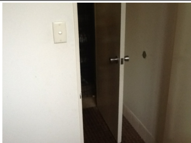
Photo No: j119922-NT0554-323 Result: Asbestos - Positive Building/Level: Main Building - Supermarket-Ground Level Room/Location: Toilets-East Feature/Material: Wall Lining-Insulating Board
