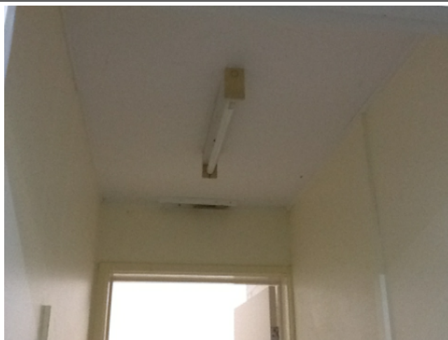
Photo No: j119922-NT0554-331 Result: Asbestos - Positive Building/Level: Main Building - Anglicare-Ground Level Room/Location: Connecting passage-Throughout Feature/Material: Ceiling-Compressed Cement Sheet
