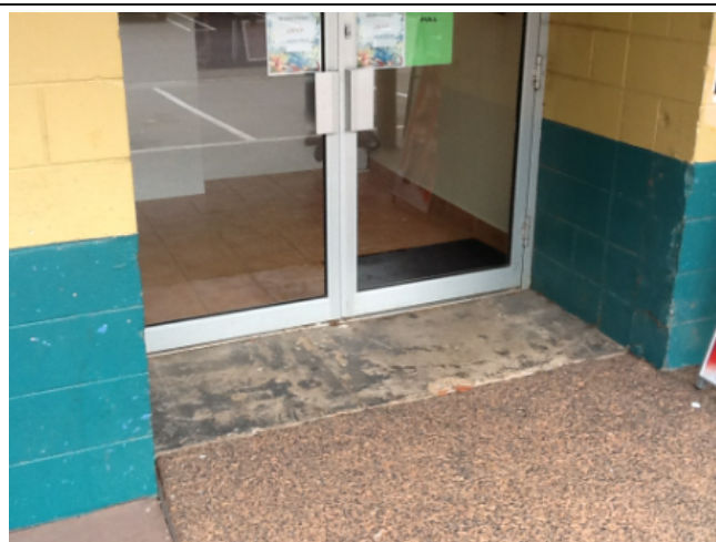
Photo No: j119922-NT0554-339 Result: Asbestos - Presumed Positive Building/Level: Main Building - Darwin Midwifery Group-Ground Level Room/Location: Exterior-North Feature/Material: Floor-Adhesive
