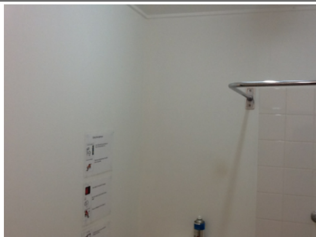
Photo No: j119922-NT0554-332 Result: Asbestos - Positive Building/Level: Main Building - Anglicare-Ground Level Room/Location: Female Toilets-North & West Feature/Material: Wall Lining-Insulating Board
